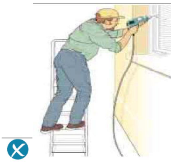
Incorrect – steps side on to work activity
