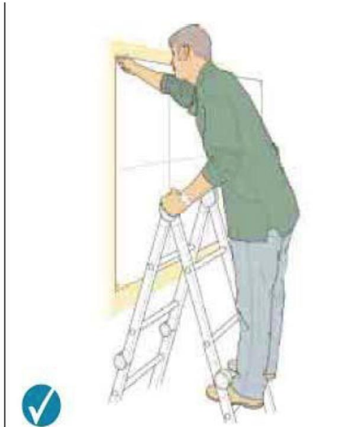
Correct – two clear rungs. Don't work any higher up this type of stepladder.
