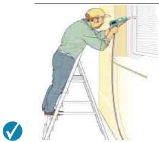
Correct – steps facing work activity
